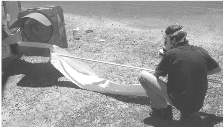
Fig. 6- probing AIP Blanket formulation into the aeration duct/phosphine reaction chamber
